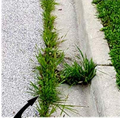
Pull these weeds from the gutter and in between the road and the gutter.
